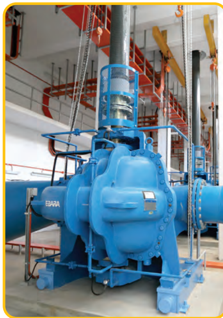
Typical installation of VDM pump with vertical shafting.
