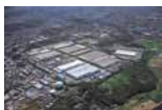
Fujisawa Plant, JAPAN
